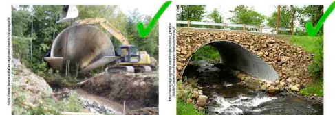
The installation of an open bottom corrugated metal culvert.
